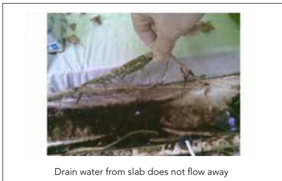
Gutter with rough surface Need some acid for cleaning
