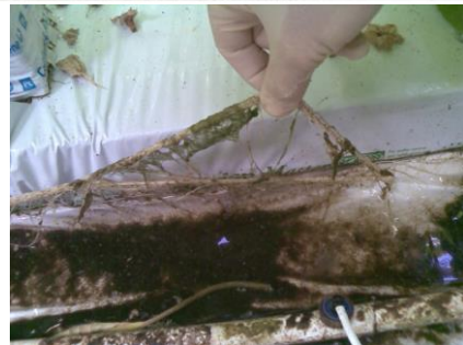
Drain water from slab does not flow away
