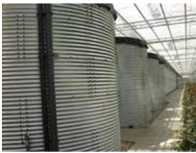
Empty silo's, sludge out, and disinfect
