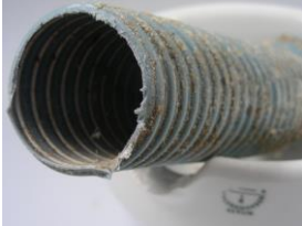
Tube to drainsystem Difficult to reach
